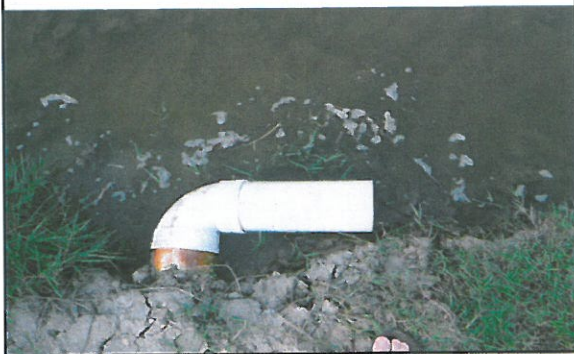
Additional pipes installed in Pond 17
